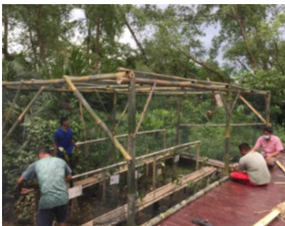
Safety Fence Installation to protect mangrove
